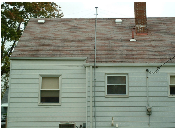
Antenna mounted against the house
