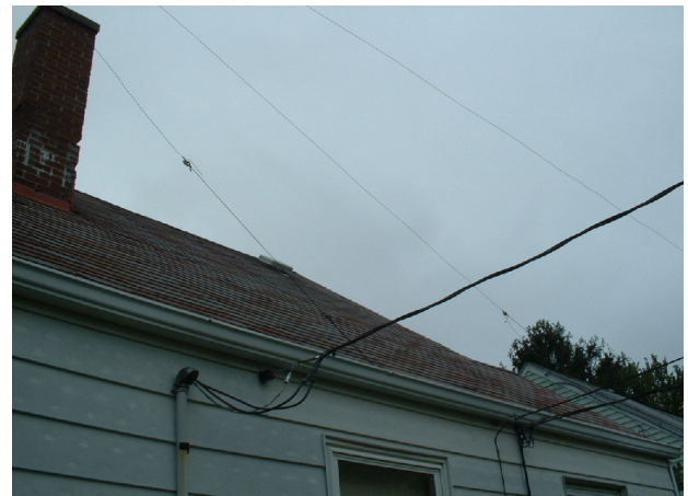
Dipole tie off. Top to bottom is 40-20-10.
