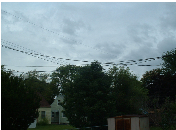
Power, cable, telephones lines crossing backyard
